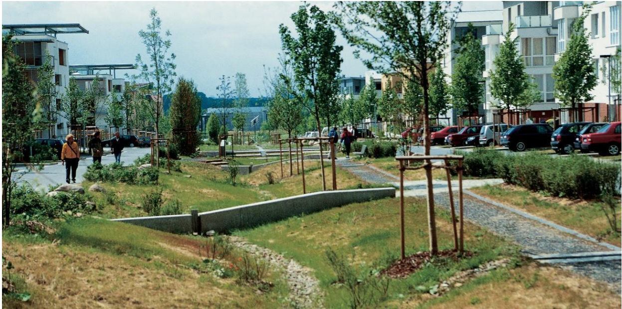
Figure 4.4 Bioswales, Kronsberg (Hannover) – Germany
