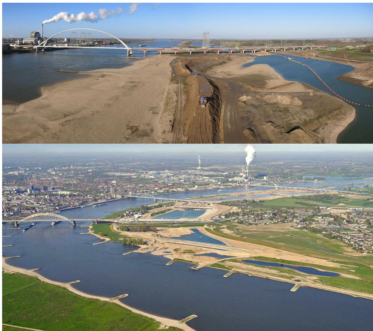
Figure 4.5 The Room for the Waal Project during (above) and after its completion (below) (Nijmegen) – the Netherlands
