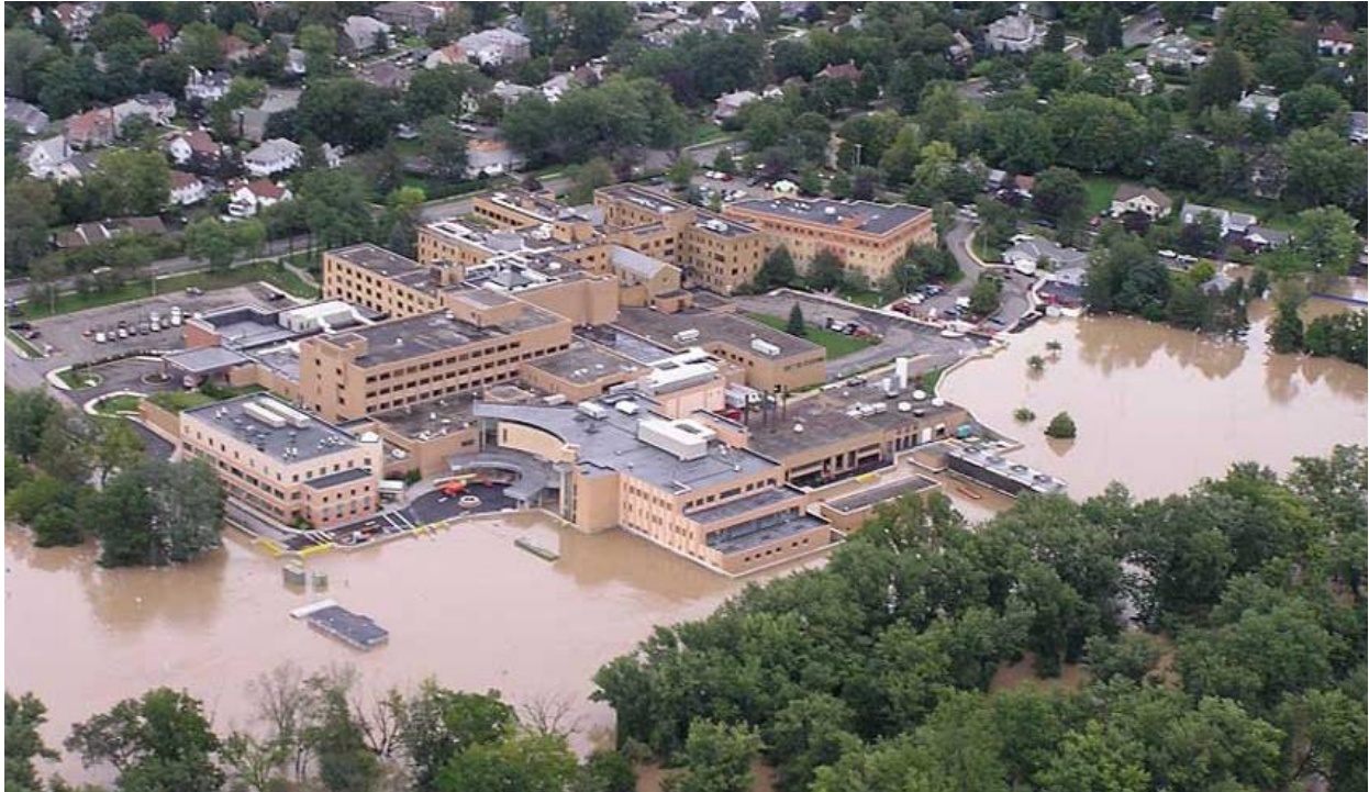
Figure 1.2 Floodwall protecting Our Lady of Lourdes Hospital during Tropical Storm Lee in September 2011– Binghamton (New York), US
